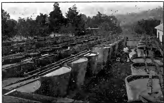
Unique Concrete Crystallizing Vats at Asti.
